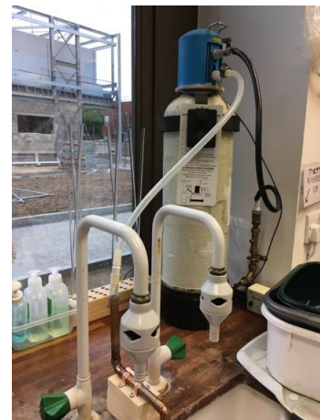
Fig 11: Distillation equipment in a school lab requires a double check valve on the supply
