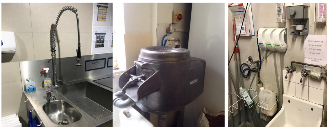
Fig 12: examples of equipment typically found in school kitchens
